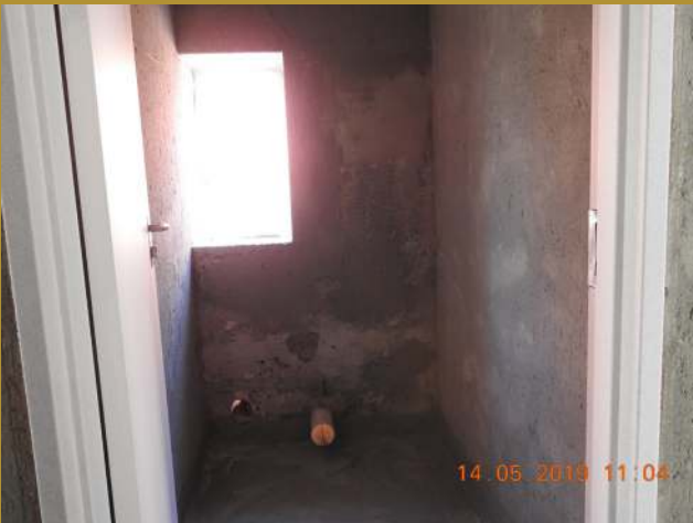
Bathroom renovations, doors, frames and new plumbing
