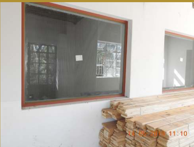
New safety glass and frames, plastering and painting
