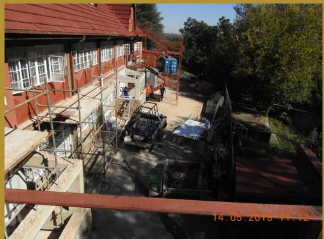
External replacements including window repairs, plastering, etc.
