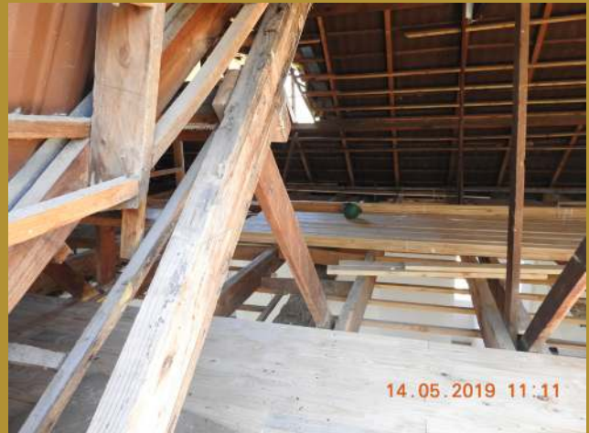
Floor replacement of lofted rooms
